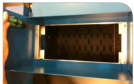
Figure 4. Installing Second Frame Tab
